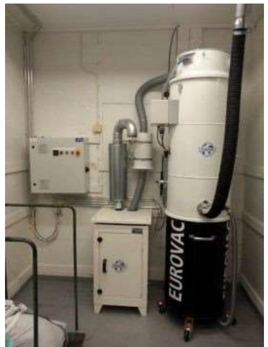
Eurovac-filtering unit with 200 l tank
