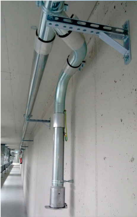
Central vacuum pipeline
