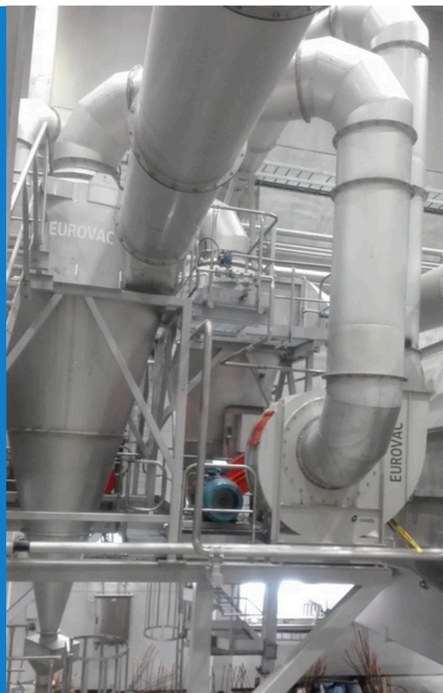
Eurovac cyclone as part of an industrial dust extraction system
